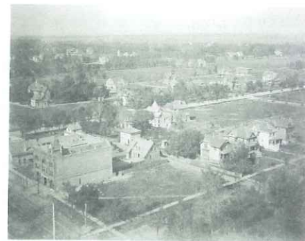
Ridgeland, 1896, looking northwest from Cuyler Ave. and Lake St.
