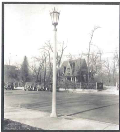
A view of the Austin home. The gate is at the far left. (Photo donated by Dwight Austin)
